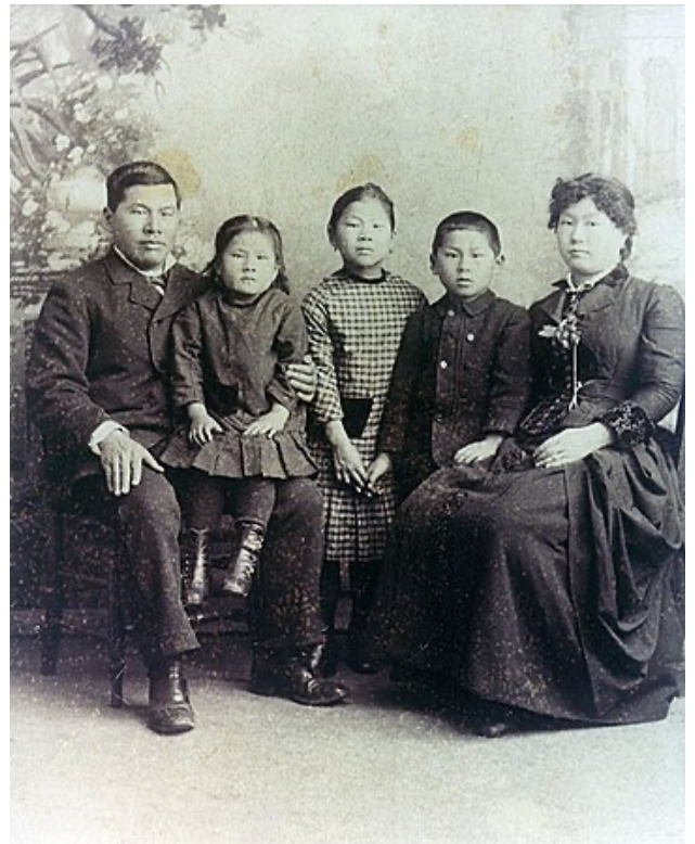
The Tape family: Photo from “The Tapes of Russell Street: An Accomplished Family of School Desegregation Pioneers,” by Daniella Thompson, BAHA, April 30, 2004.
